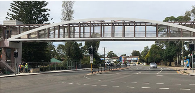
Starkey Street Pedestrian bridge, Forestville, NSW
